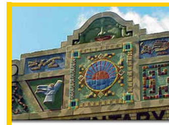
The snakes sculpted by Luis Lopez (1928) gave Bowie School its nickname, La Escuela de las Viboras (the school of snakes). The unique façade features blending Mexican motifs such as Toltec feathered headdresses, Aztec heads, and Quetzlcoatl, Mexico's fabled feathered serpent.
